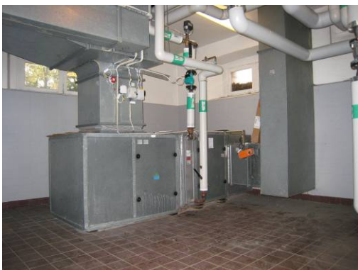
Tilluftsaggregat TA1.
